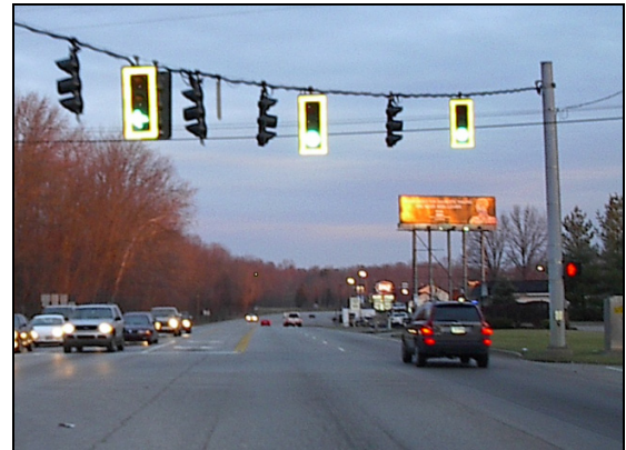
Figure VI-11. Retro-reflectorized Signal Back plates at US 31W and KY 1638 in Muldraugh
