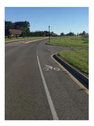
5) Roadway Shoulders are the part of the roadway that is adjacent and contiguous to the regular travel lanes. This portion of the roadway can be used by bicyclists. Paved shoulders can be an appropriate bicycle facility along roadways that do not have curb and gutter but have open drainage.
